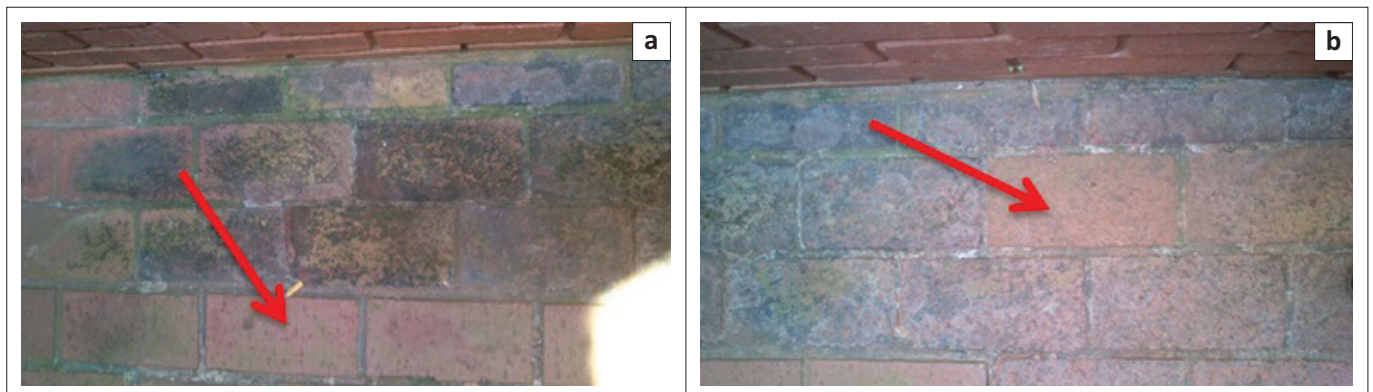
FIGURE 4: Some (a) pavement bricks with no presence of algae and some (b) pavement bricks with the presence of algae (pointed by red arrow).
