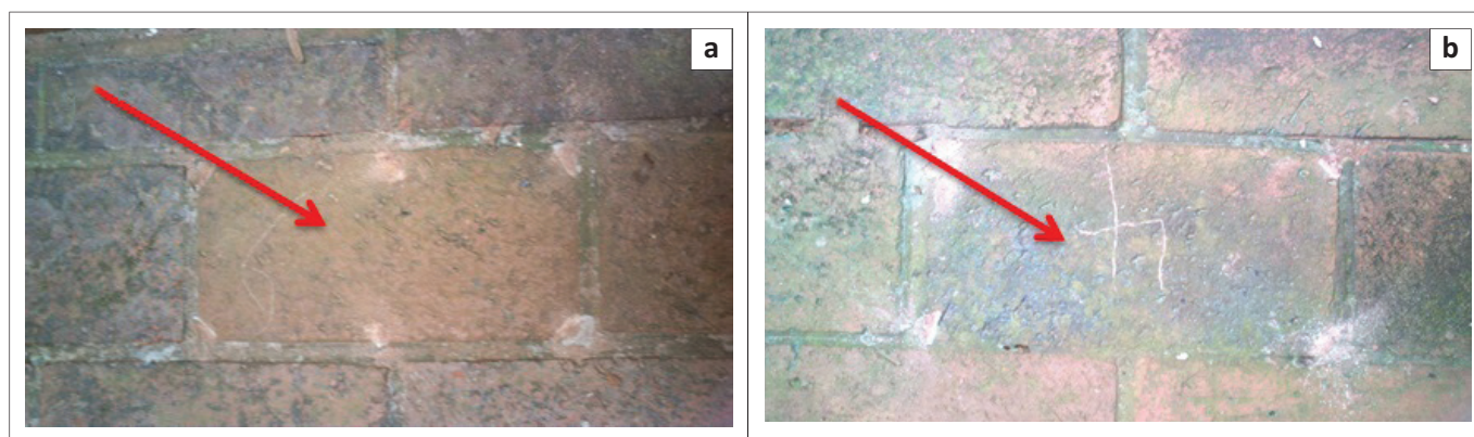
FIGURE 5: (a) Pavement brick with minimal presence of algae and (b) pavement brick with high levels of algae
