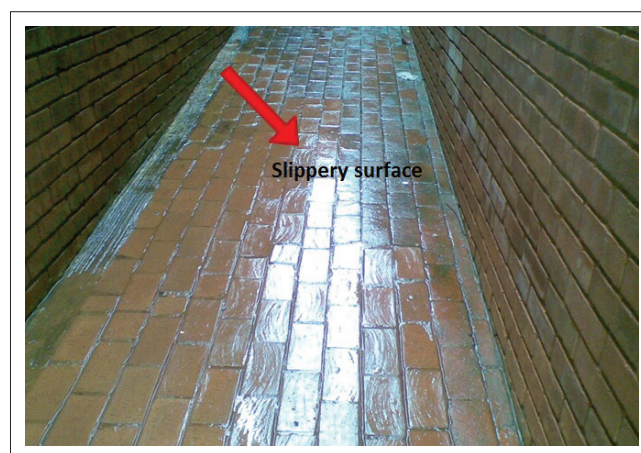
FIGURE 1: Algae growing on a building's wall and pavement.
