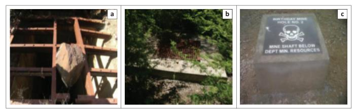
FIGURE 3: Shaft-closing structures at Sutherland goldfield: (a) heavy steel grate, (b) steel wire screen and concrete and (c) concrete plugs with landmark.
