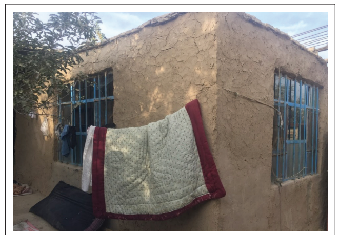
FIGURE 4: A single-storey mud brick masonry house with a flat roof.
