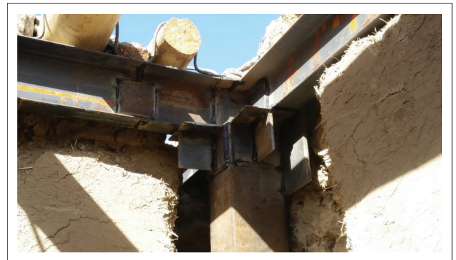
FIGURE 15: Splice in beam.
