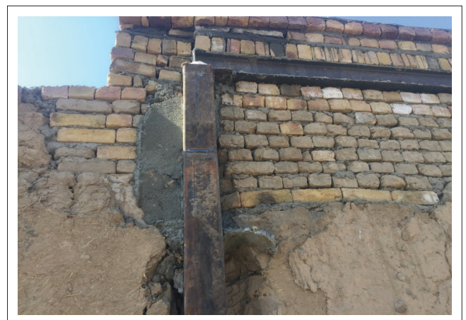
FIGURE 16: Splice in column.
