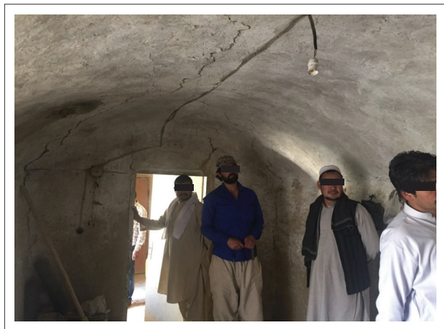
FIGURE 5: A single-storey mud brick masonry house with a barrel-shaped roof.
