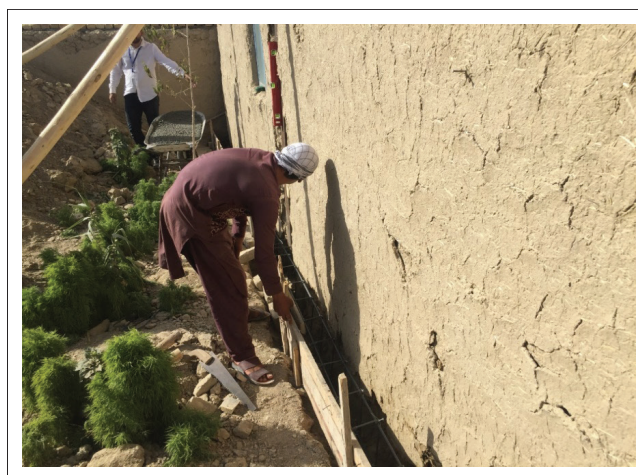
FIGURE 6: Implementing an additional RCC foundation ring.
