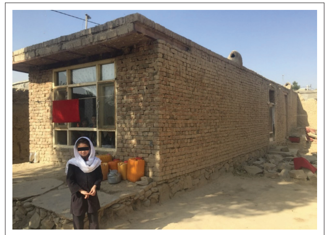
FIGURE 3: A single-storey burnt brick masonry house with a flat roof.
