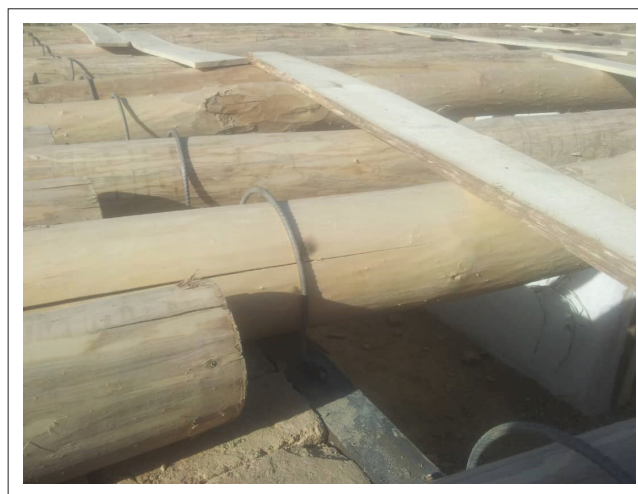
FIGURE 9: New roof cover and its connection with horizontal ties.
