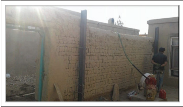
FIGURE 12: Installing buttress for surrounding wall.
