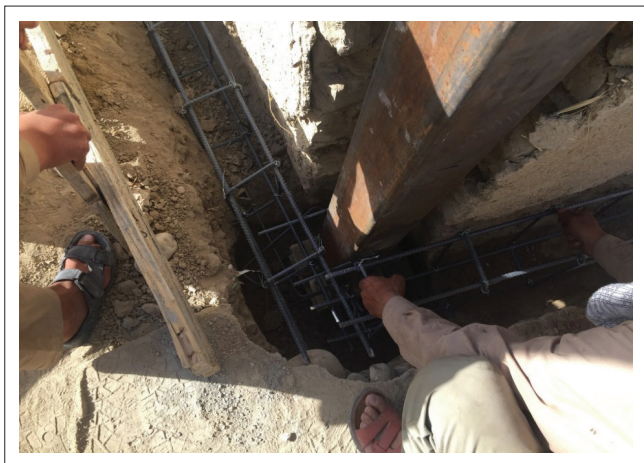
FIGURE 7: Placing vertical tie inside the foundation ring.
