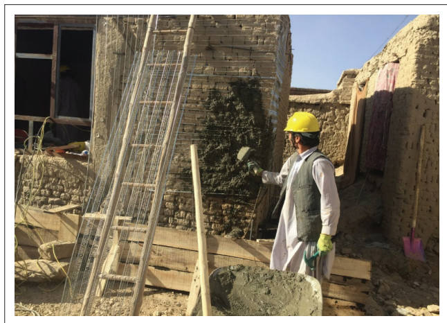
FIGURE 10: Wall mesh and plaster.
