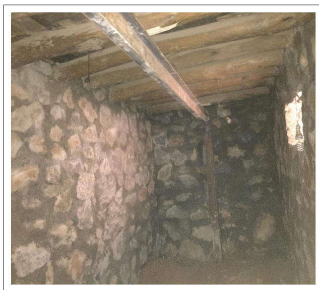
FIGURE 11: Additional stone masonry for basement improvement.
